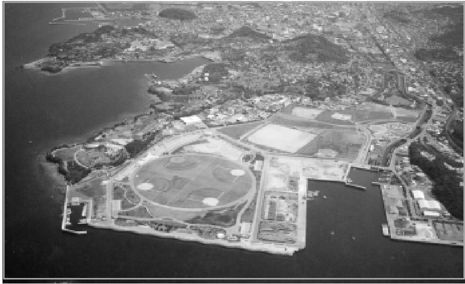
Minamata Bay Reclaimed Land (Eco Park Minamata)
