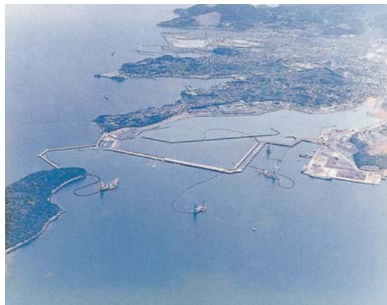
Dredging using a Cutterless Pump Dredging Ship
